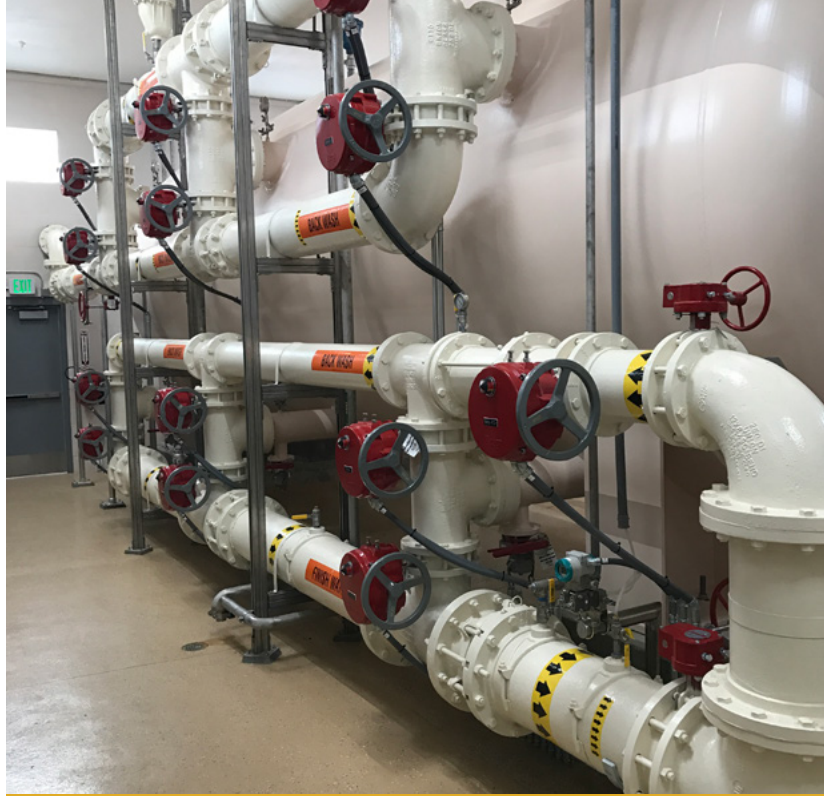
New Well 27 Treatment Facility
