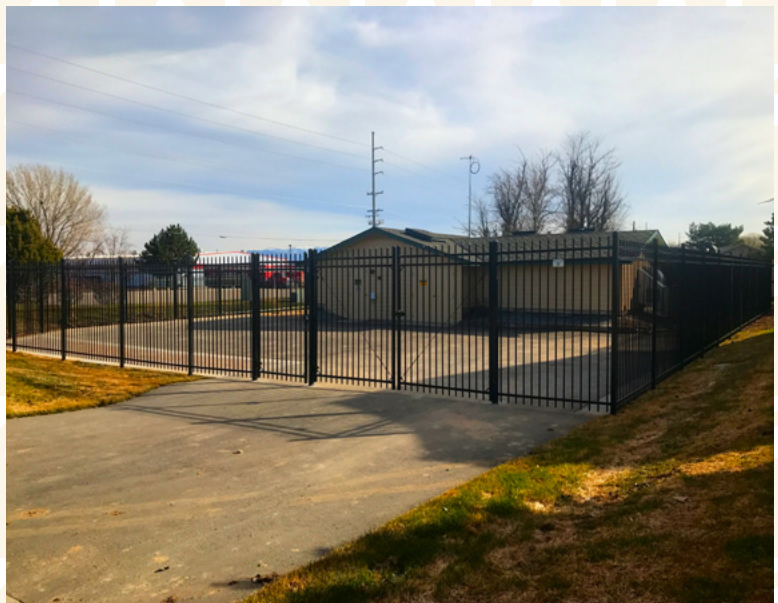
Well 14 Production Facility
