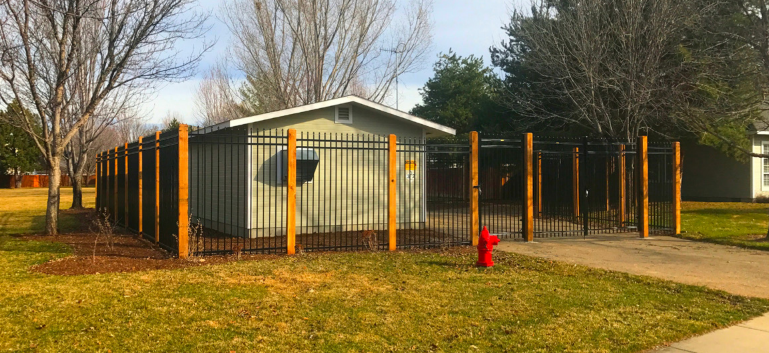
Well 18 Production Facility
