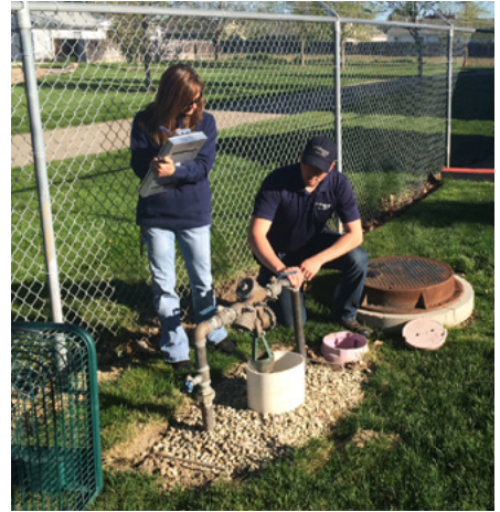
Meridian inspectors testing a backflow prevention assembly.
